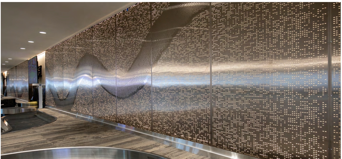
Feature wall: backlit panels in Fused Nickel Bronze with Satin finish, custom Eco-Etch pattern and custom perforation pattern
